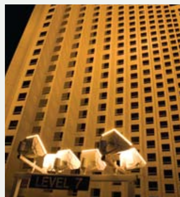
FIGURE 14. High pressure sodium exterior structure lighting of a building
