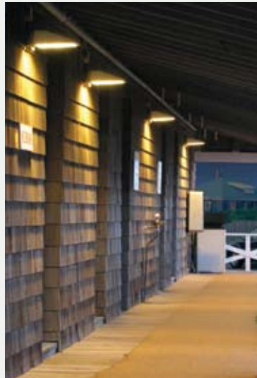
FIGURE 8. Scheduled group relamping has proven to be more cost effective than spot relamping.
